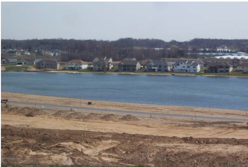
An example of the type of neighborhoods being constructed in Byron Township
